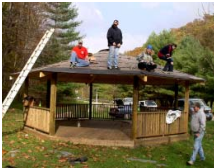
Volunteers construct gazebo at Community Center
